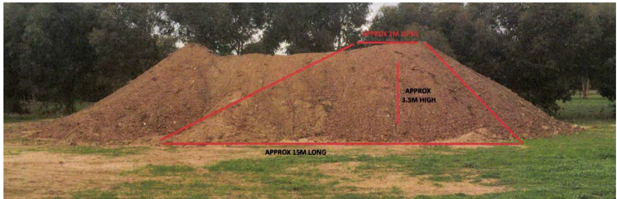
Earthen mound during construction – showing eventual size with red lines
