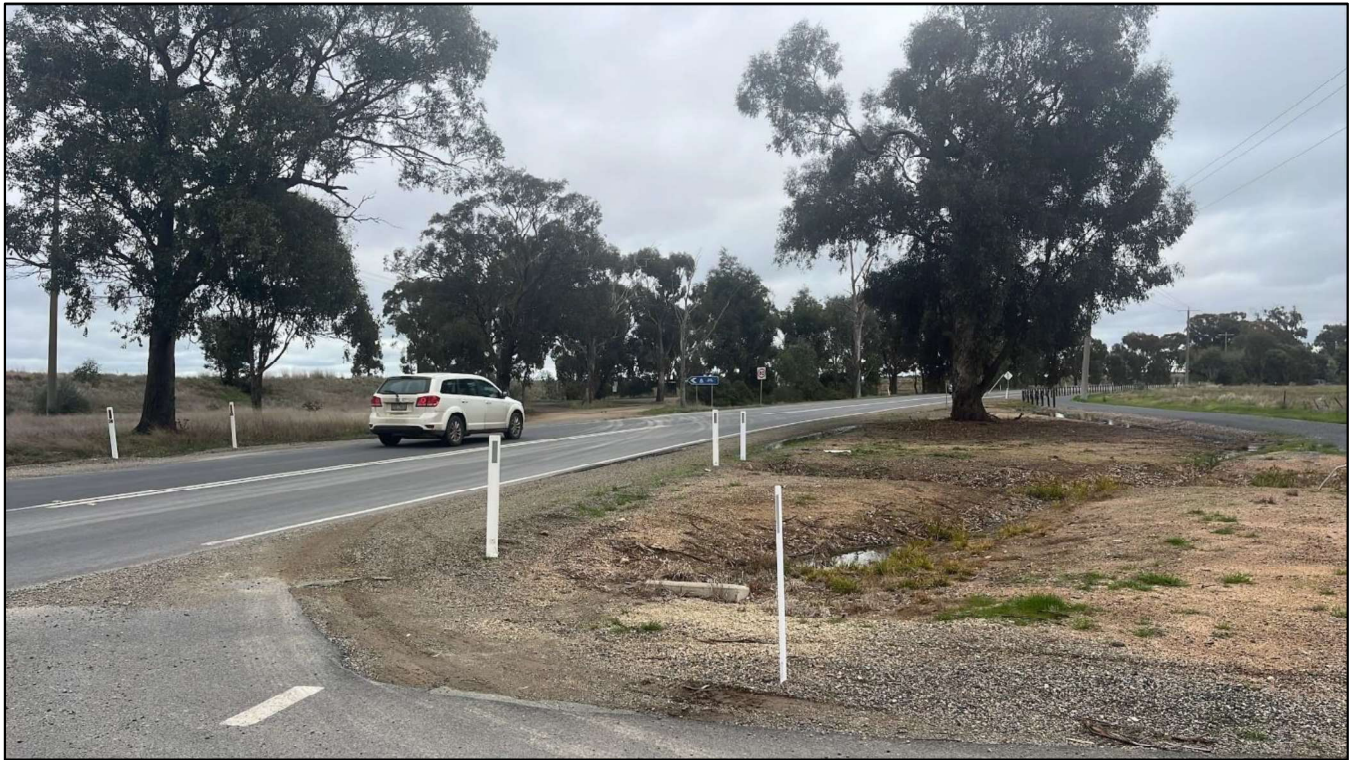
Figure 12: Sight distance along Murray Valley Highway from Brears Road - view west
