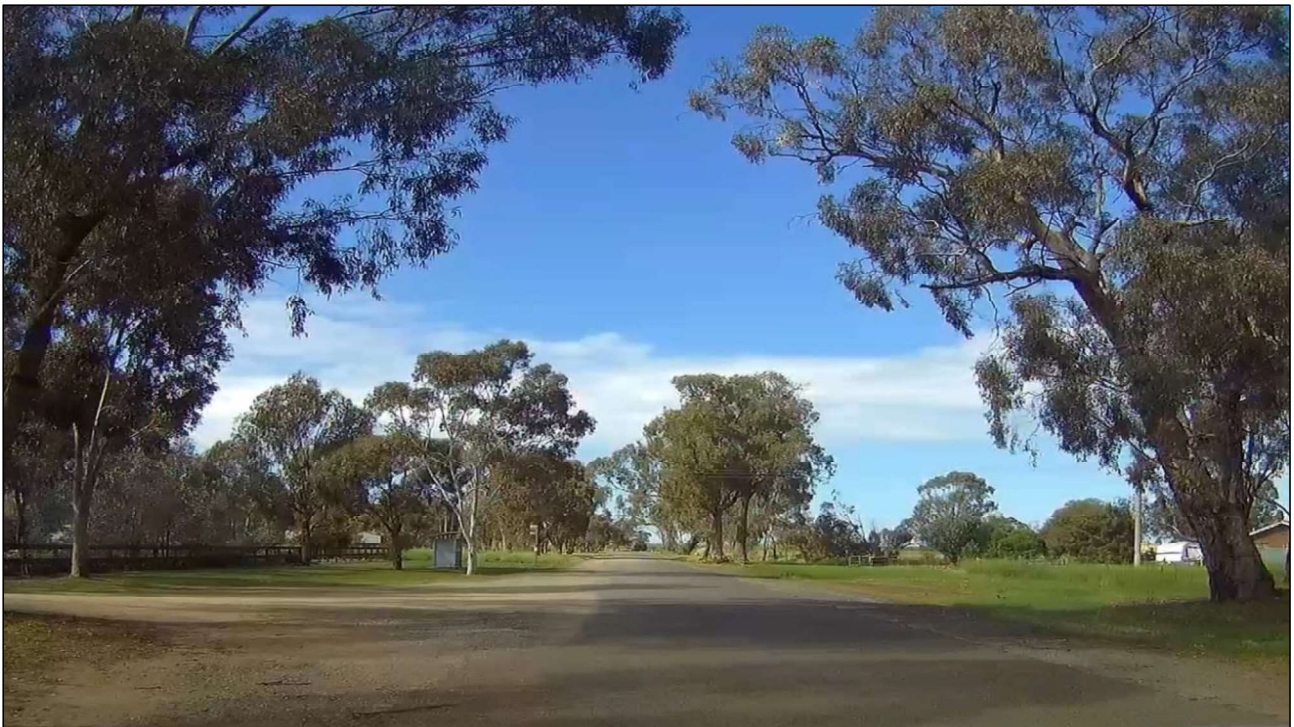
Figure 6: Brears Road looking south, the caravan park access and a bus stop to the left
