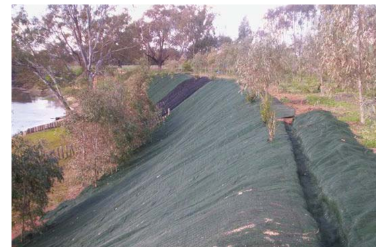
Soft engineering (geo-textile matting) example
