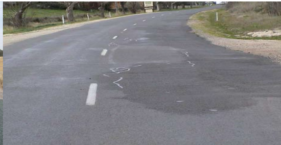
Condition 6 Moderate failures and shape loss
