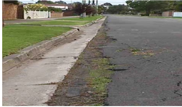
Condition 6 - Movement and Concrete breakdown
