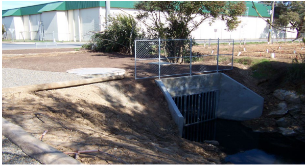
Condition 0 - As new condition
