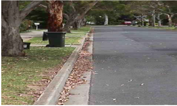
Condition 3 - Old but only Minor loss of shape & movement
