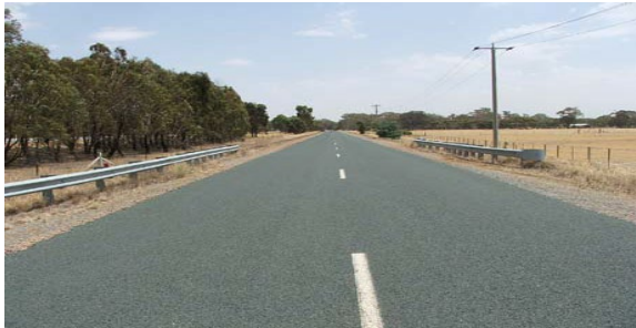
Condition 0 – 1 No Failures no Shape loss
