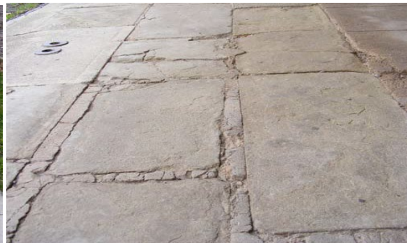
Condition 7 - Extensive cracking and movement
