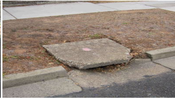
Condition 7 - Poor overall condition
