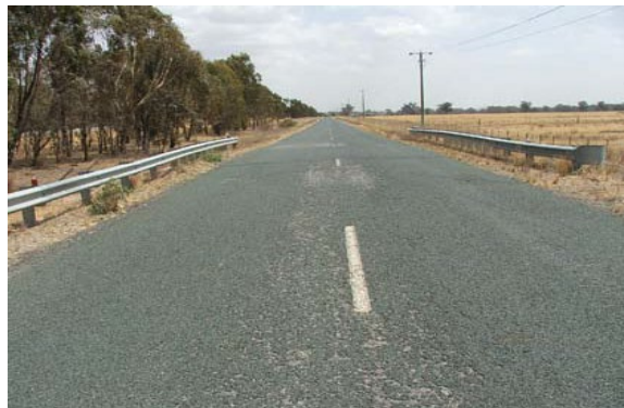
Condition 6.5 - 7 Oxidized and Stripping
