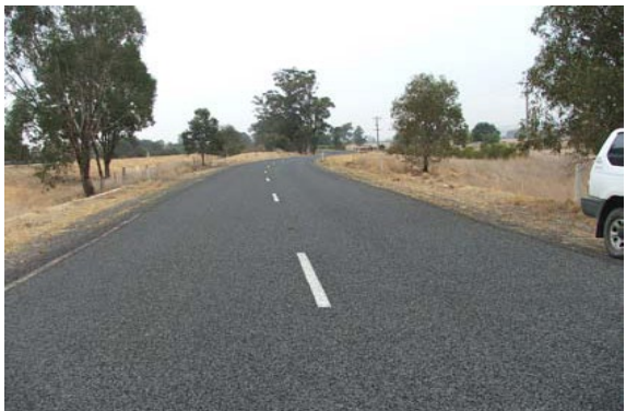
Condition 0 – 1 Seal in Excellent near new condition
