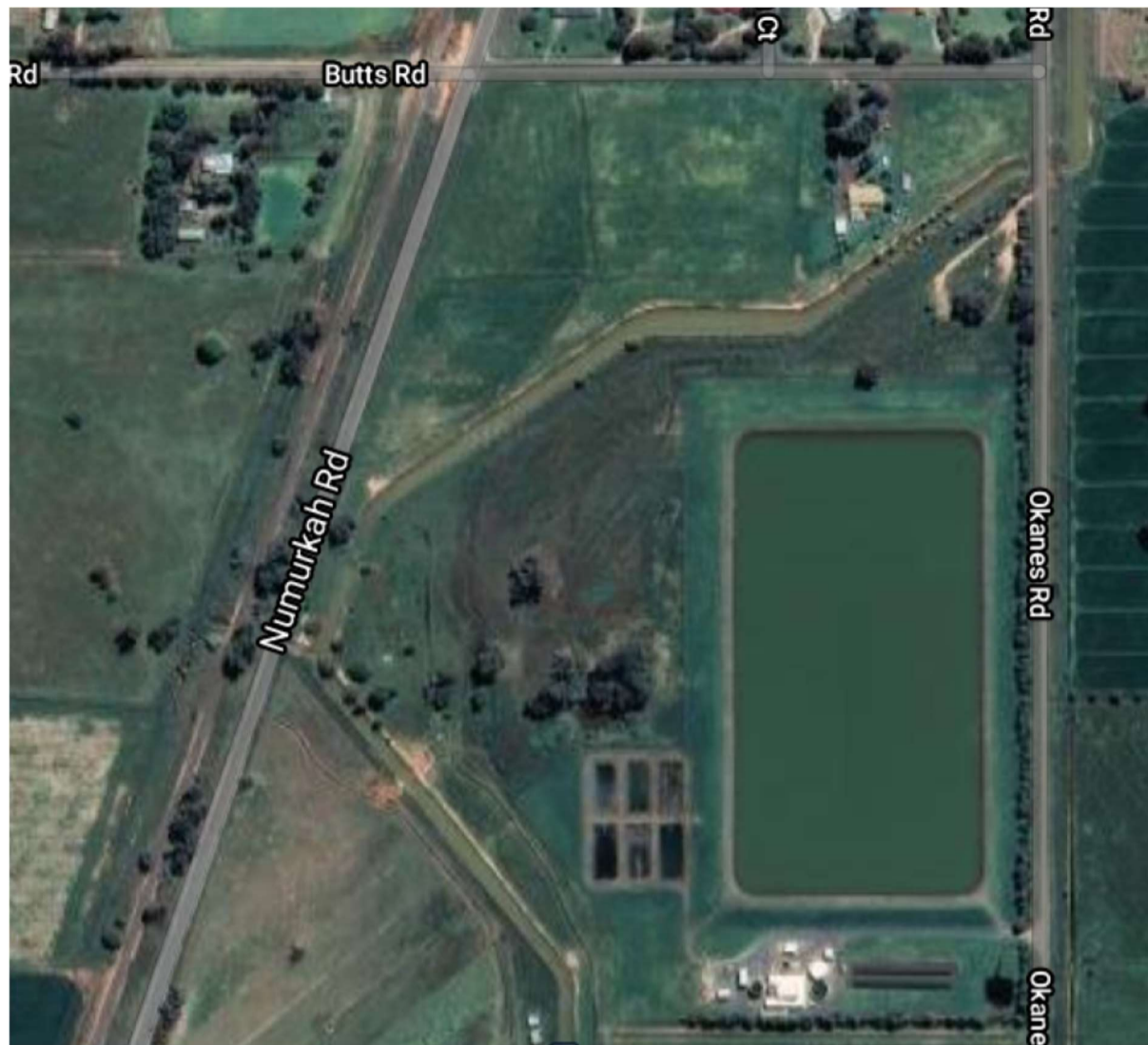
Goulburn Valley Water Facility
