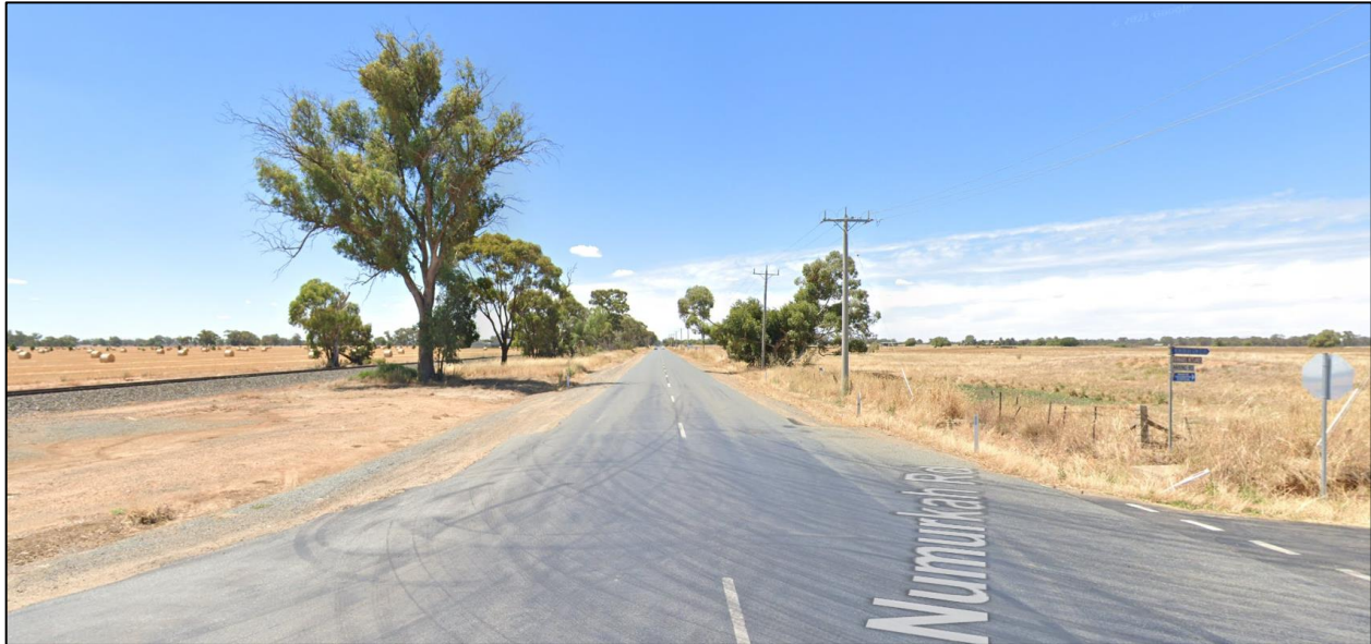
Figure 4 Numurkah Road/Tocumwal Road/Naring Road Intersection facing north
