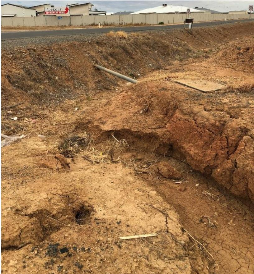
**Figure 10.** Botts Road open drainage channel, characterised by unvegetated banks, undercutting and erosion, looking north-west.
