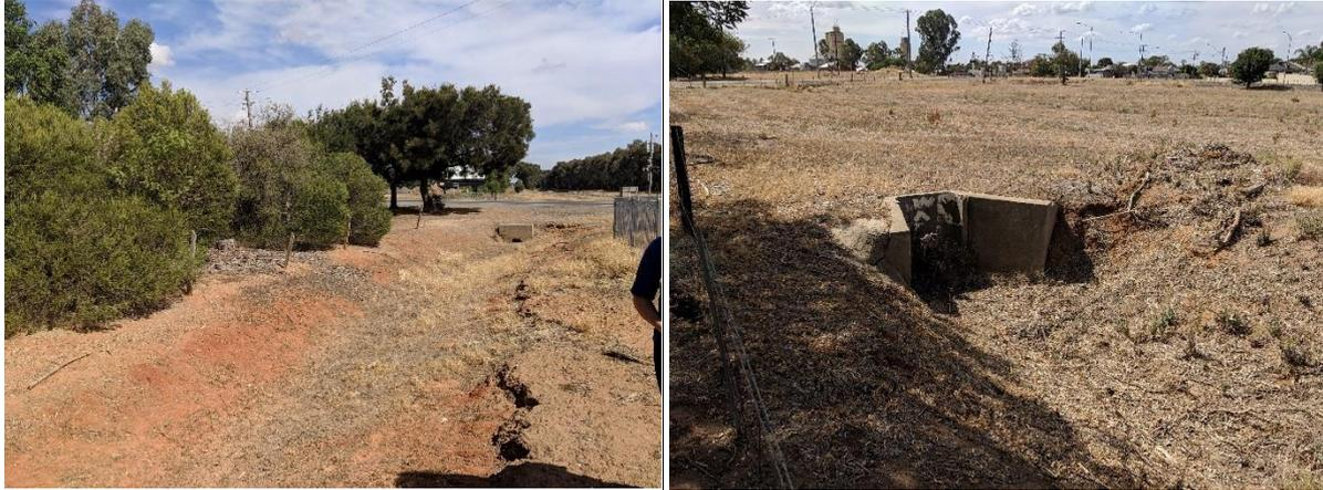
**Figure 8.** Example of typical spoon drain and blocked culvert found through the study area.
