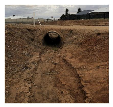
Figure 11. Culvert and streambed in Botts Road channel, looking south. Note steep, exposed banks and evidence of erosion.
