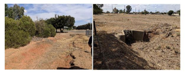
Figure 8. Example of typical spoon drain and blocked culvert found through the study area.
