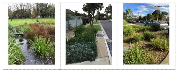
Figure 34. Street-scale biofilter examples
