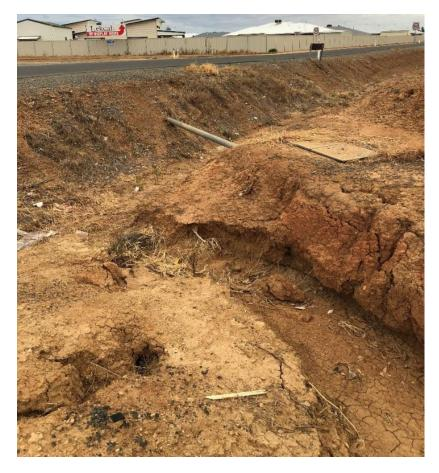
**Figure 10.** Botts Road open drainage channel, characterised by unvegetated banks, undercutting and erosion, looking north-west.
