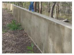
Concrete Retaining Wall Levee
