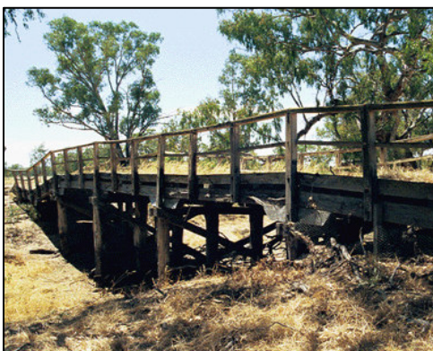
Timber bridge over Sheepwash Ck, Kotupna
