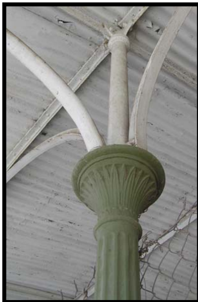
Figs 6 & 7 Railway Station building, platform, verandah, and fluted iron columns. Source: Lorraine Huddle Pty Ltd. 2005.
