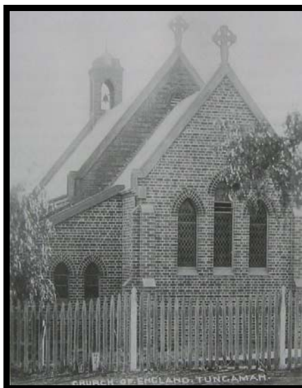
Fig 10. 1889 St Alban's Anglican Church, 8 Barr St. The Gothic design has a high degree of integrity with unpainted red brick walls and buttresses, lancet windows finials in the form of celtic crosses, and brick bell tower. Source: Lorraine Huddle 2004
