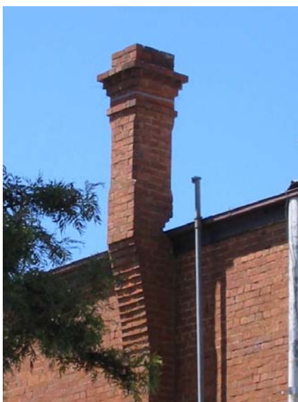
Evidence of a creative chimney-corbel craftsman. Cobram.
