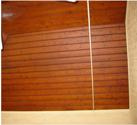
Figs 47&48. Grain store interior and exterior. The steeply raked ceiling is clad in polished lining boards and pressed zinc clad the upper wall in the unusual interior space. These are all significant features. Source: Lorraine Huddle Pty Ltd 2003.
