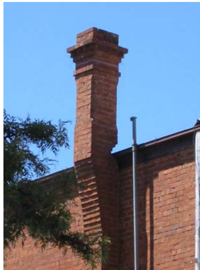
Evidence of a creative chimney-corbel craftsman. Cobram.
