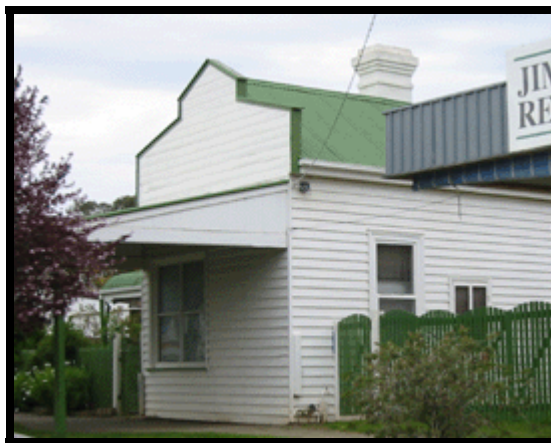
Former shop, with skillion verandah and weatherboard parapet. 19 Beek Street Katamatite. Source: Lorraine Huddle 2004.
