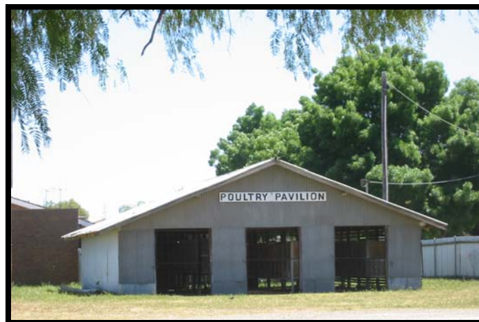
Poultry Pavilion clad in galvanised corrugated iron (not zincalume). Source: Lorraine Huddle 2004.
