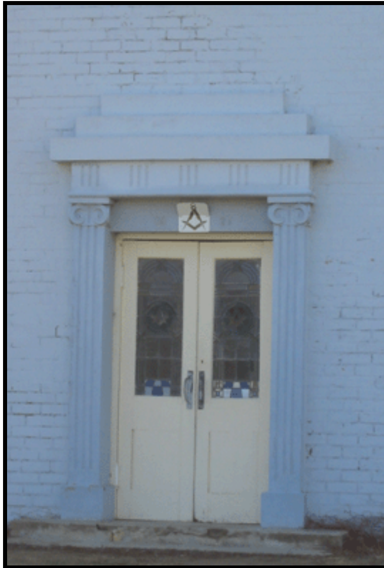
Detail of Masonic Lodge Doorway showing the classical door way with Ionic pilasters supporting a stepped pediment, and leadlight windows with Masonic symbolism.
