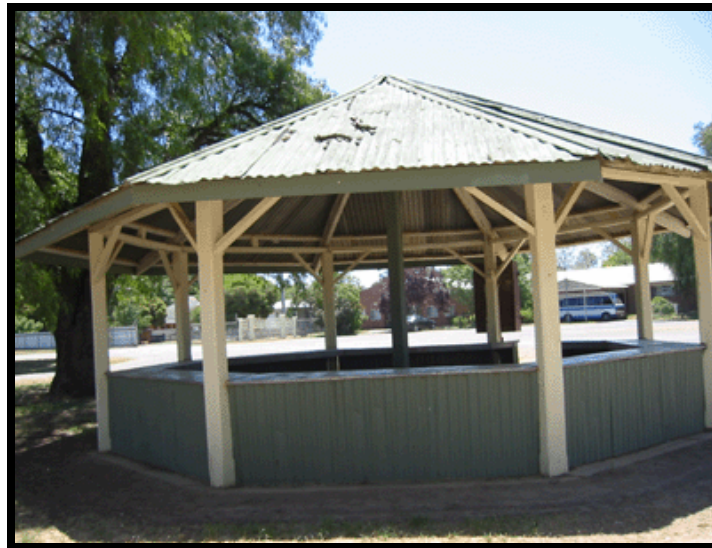
c 1909 Octagonal Pavilion of timber and galvanised corrugated iron: Source: Lorraine Huddle 2004.
