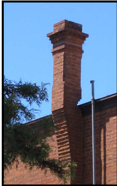
Unpainted red brick chimney with interesting corbelled method of building around the spouting. Source: Lorraine Huddle Pty Ltd 2004
