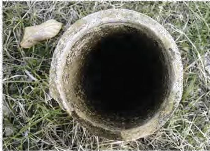
Photo 8 – View of asbestos pipe in Lot 2.
