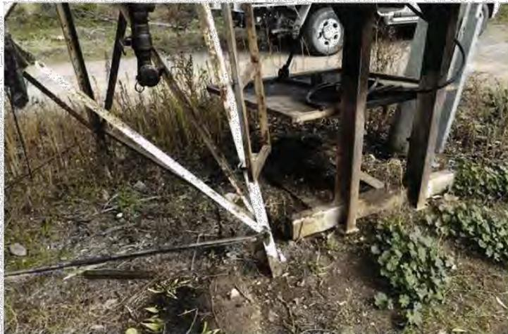
Photo 23 – View of soil staining beneath diesel AST outlet
