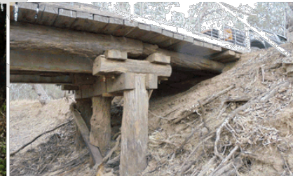
Condition 6 - Road Bridge - Fair to poor overall condition
