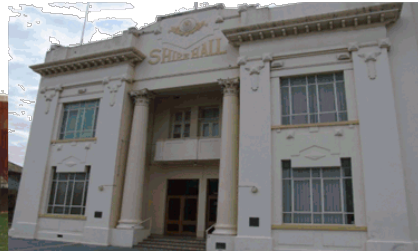
Condition 5 - Fair overall condition
