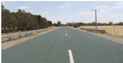
Condition 0 – 1 No Failures no Shape loss
