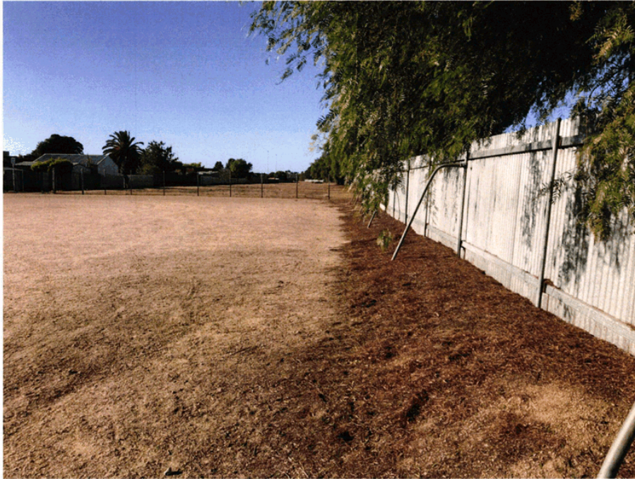
Fence currently along proposed new car park & entrance which is a tripping hazard for young children
